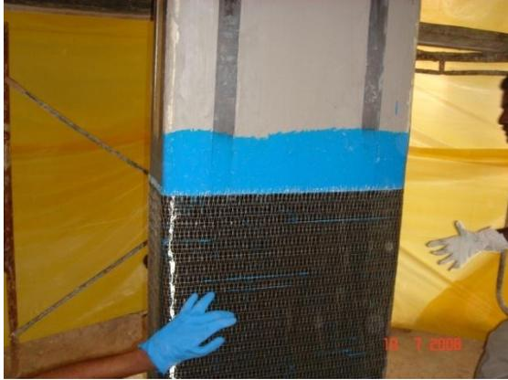
**Figure 4: Application of CFRP Sheets**
