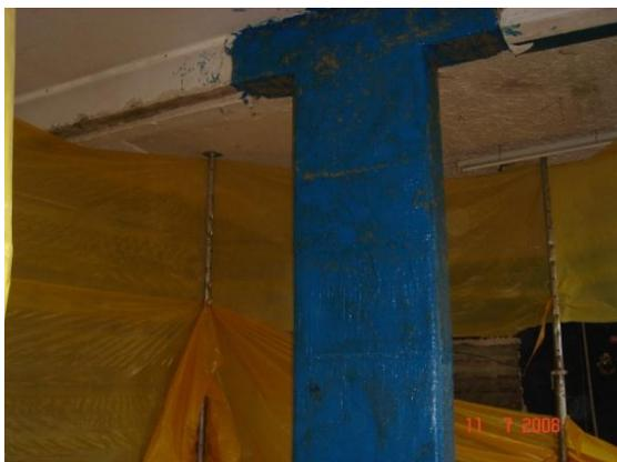
**Figure 5: Finished Column before applying plaster**
