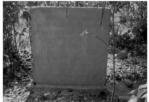
Figure 2: Constructed wall panel
