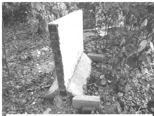
Figure 3: After laying concrete at the joint
