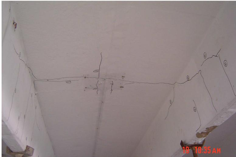
Figure 10: Cracks at T-beams flanges
