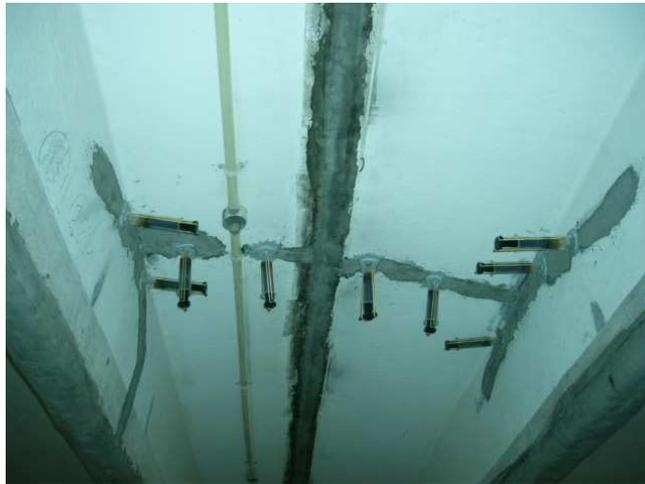
Figure 11: Repairs to non-structural cracks
