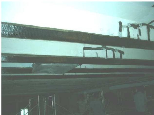
Figure 12: The beams completed with FRP work
