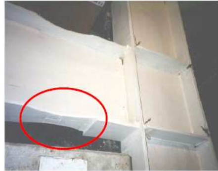
Figure 11: RBS type connection
