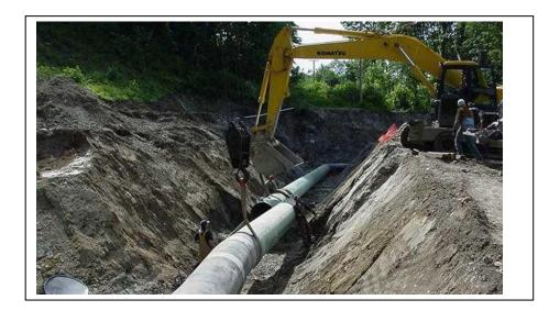
Figure 1: Typical open cut installation of buried pipelines.
