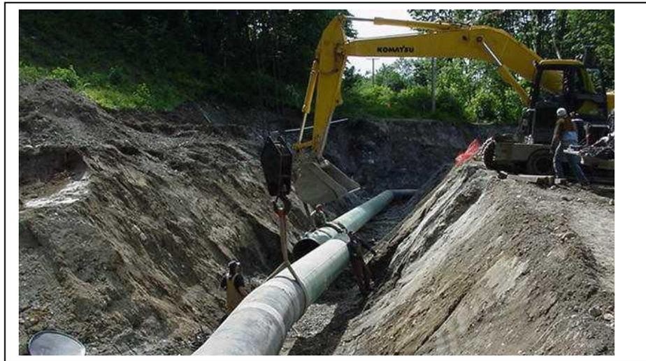
Figure 1: Typical open cut installation of buried pipelines.
