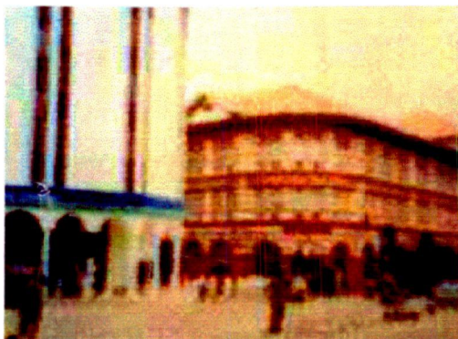
Fig.36: Violation of horizontally Grindlays Bank
