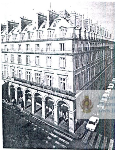
Violation of Corner Treatment
