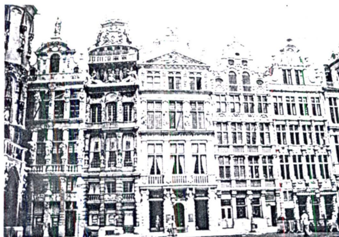
Fig. 23 Incorrect separation of floor to floor height violates the streetscape
