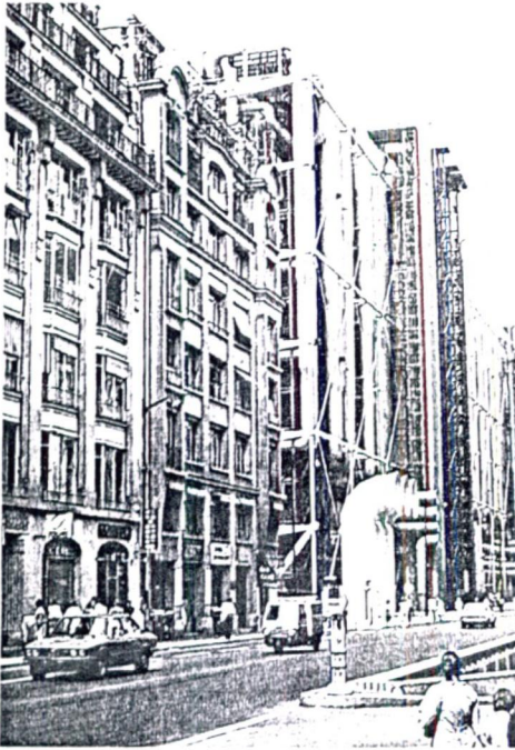
Fig. 27 Mismatch of building components
