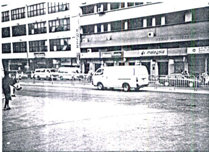
Fig. 103 Violation of Unity – Hemas and Bristol Buildings
