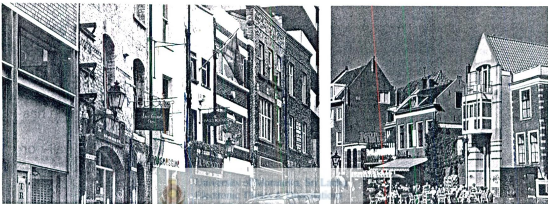
Miss match of building components violate the continuity
