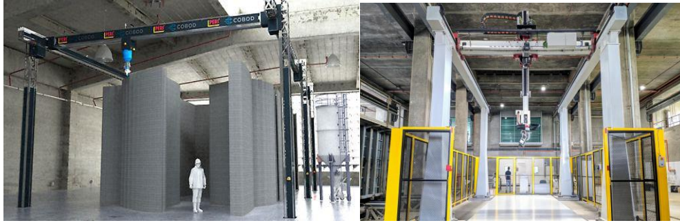
Figure 1: 3D Concrete Printing Applications in Building
