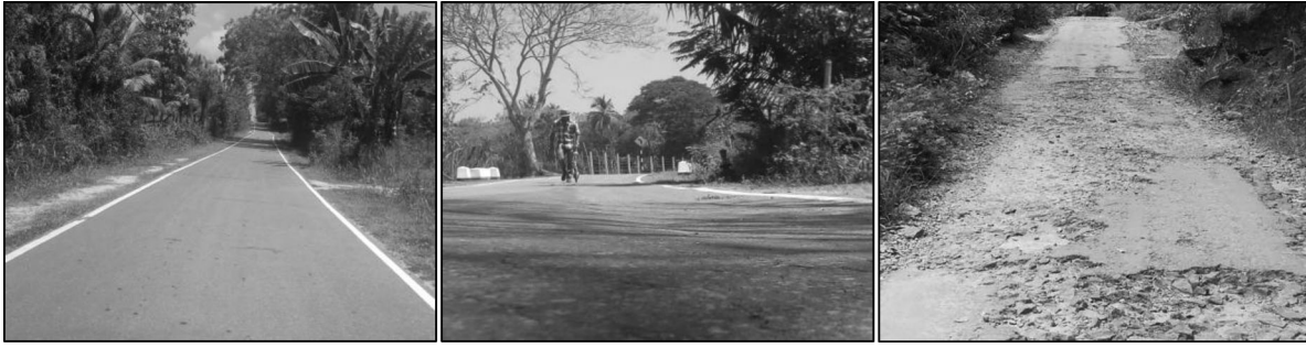
Figure 2. Example of road sections with different distress levels in rural road network.
