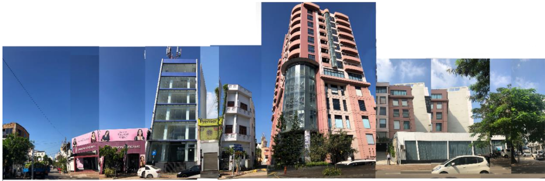
Figure 4:35: Duplication Road – sea side (Bottom of Joseph Lane) in 2021 Source: Handuni Munasinghe
