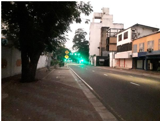
Figure 4:42: poor lighting along streets Source: Author
