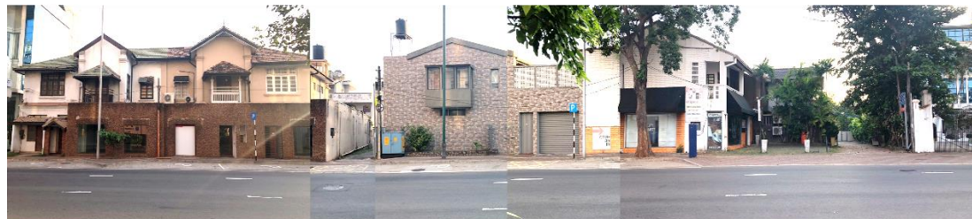
Figure 4:37: Duplication Road- land side opposite bottom of Joseph Lane in 2021 Source: Handuni Munasinghe
