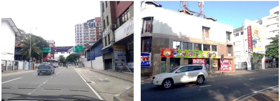
Figure 4:26: Unattractive building facades Source –author
