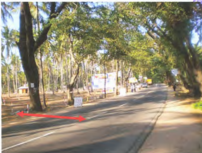
Figure 5.3 Violation of street line reservations (Ref.annex. KU 3)
