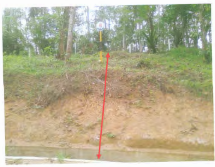
Inappropriate Plot size (Reff. Annex.KA1)
