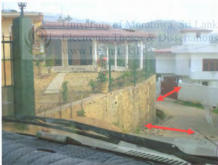
Encroachment of building lines
