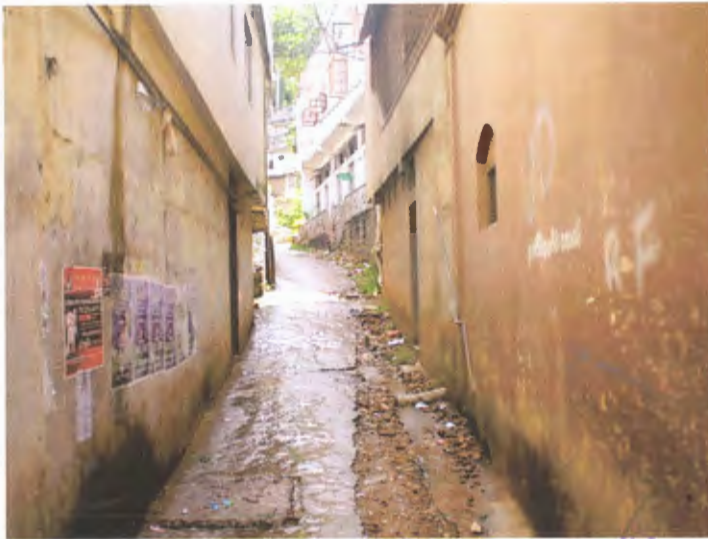
Violation of side space in hilly area
