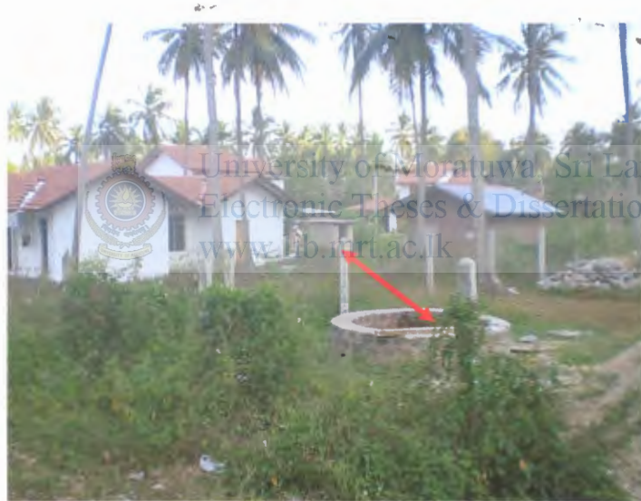
Figure 5.7 Close distance between well and septic tanks
