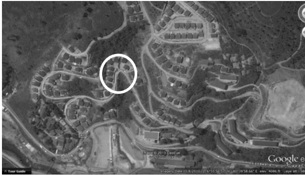
Figure 2: Location of selected houses -Google map – Upper Kothmale hydropower project Housing scheme
