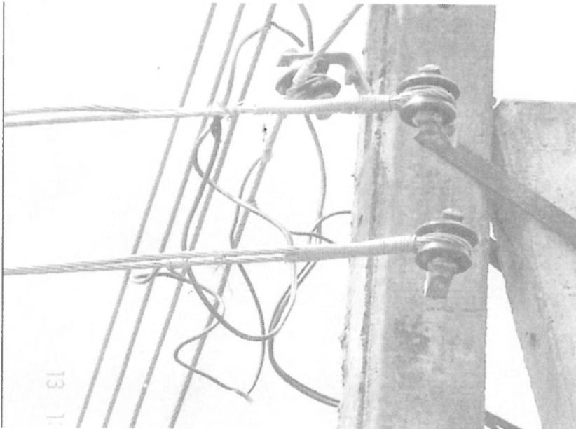
Bad jumpers increase the resistance of LT lines.
