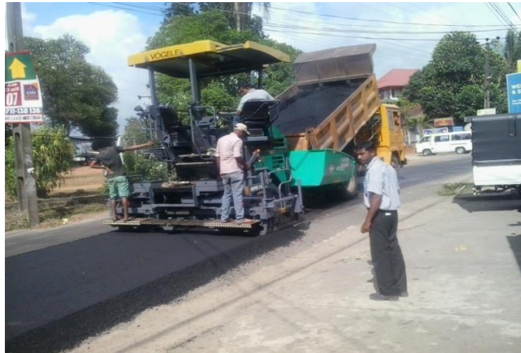
Figure 5. 5 Asphalt laying on ABC base
