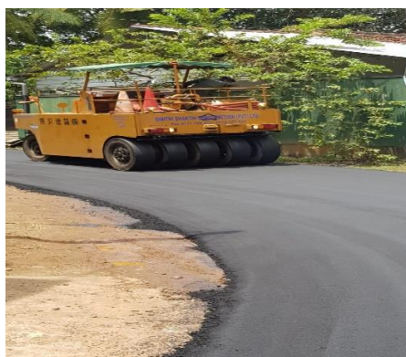
(c) Pneumatic roller
