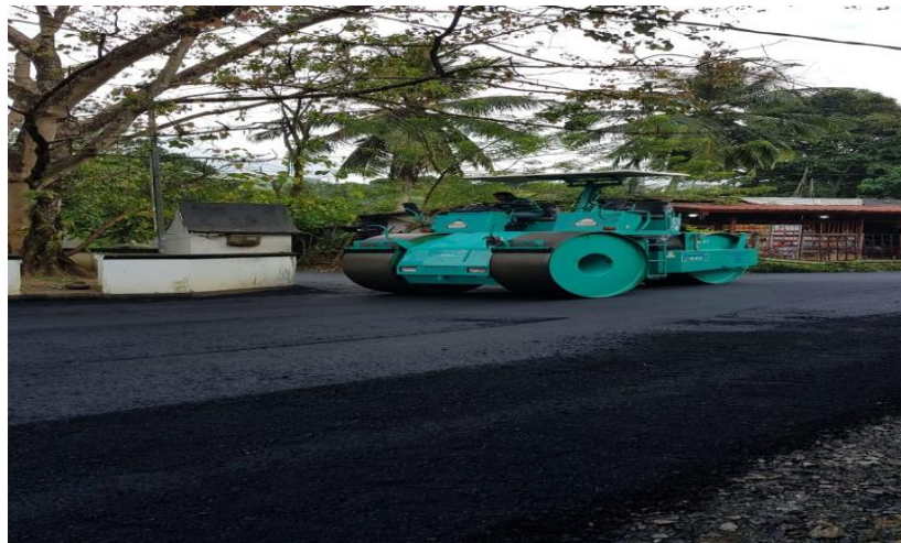
(b) Tandem wheel roller
