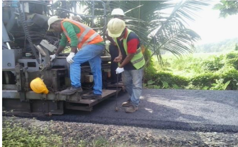
(a) Asphalt paver
