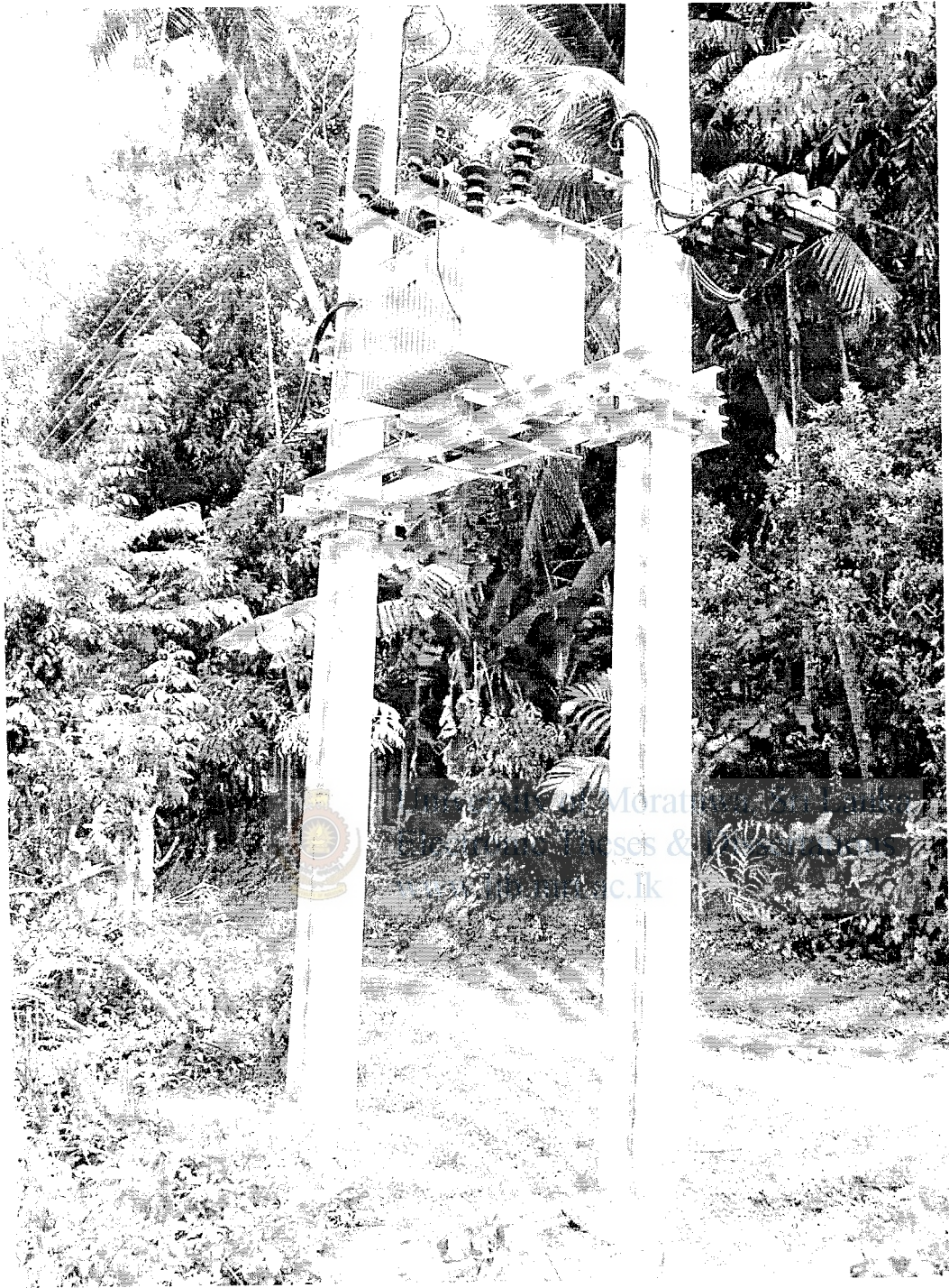
Figure 1.1 Distribution Substation
