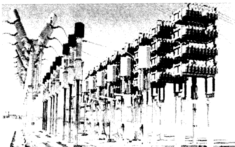
Figure 2.3: Typical stacked rack Capacitor bank
