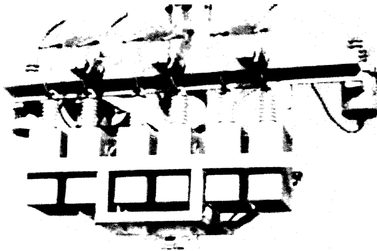
Figure 2.4: Typical pole tip mounted Capacitor bank
