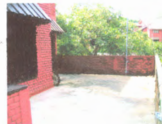
Fig. 38 Entrance court in second floor
