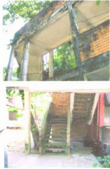
Fig. 46 – Space among the columns
