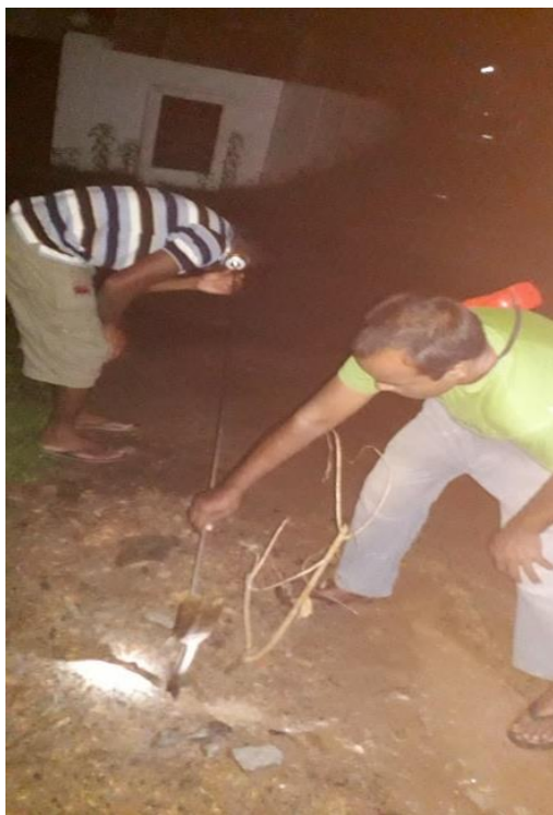
Figure 5.17 : Detection of Underground leak
