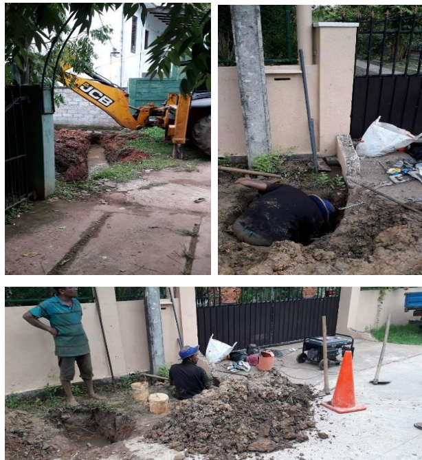
Figure 5.19 : Repair of leakage
