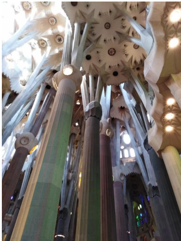
Figure 2.12: Slender columns supporting the thrust of the domed roof and towers in La Sagrada Familia, Barcelona.
