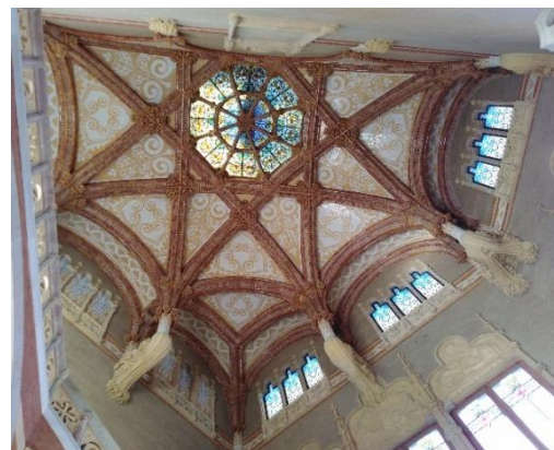
Figure 2.15: Roof structures at Hospital Sant Pau in Barcelona, indicating influence from Persian Architectural technique of Karbandi.
