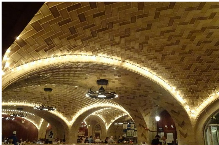
Figure 2.16: Guastavino vaulting in Grand Central Terminal, New York.
