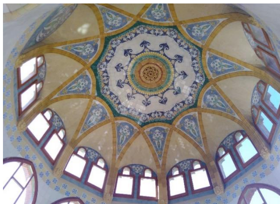
Figure 2.15: Roof structures at Hospital Sant Pau in Barcelona, indicating influence from Persian Architectural technique of Karbandi.
