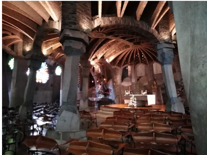
Figure 2.13: The compression only support structure of the Crypt at Colonia Guell.
