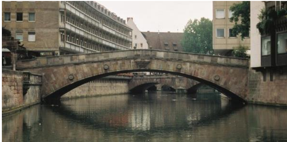
Figure 2.8: Fleisch Bridge, Nuremberg. Source: Structurae.net/ photographer: Nicolas Janberg.
