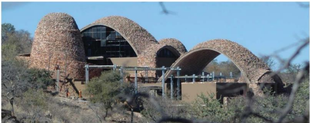
Figure 2.50: Mapungubwe National Park visitor centre. Source: Ramage et al. [18]
