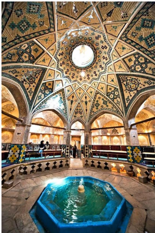
Figure 2.10: A Karbandi structure in Zoltan Mir Ahmad – a traditional Persian bath- in Kashan, Iran. Image courtesy: Mostafa Aref Hagi.
