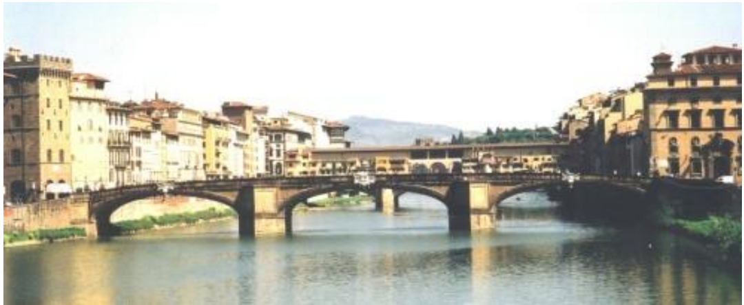
Figure 2.7: Ponte Santa Trinita. Source: Structurae.net/ photographer: Karl Gotsch
