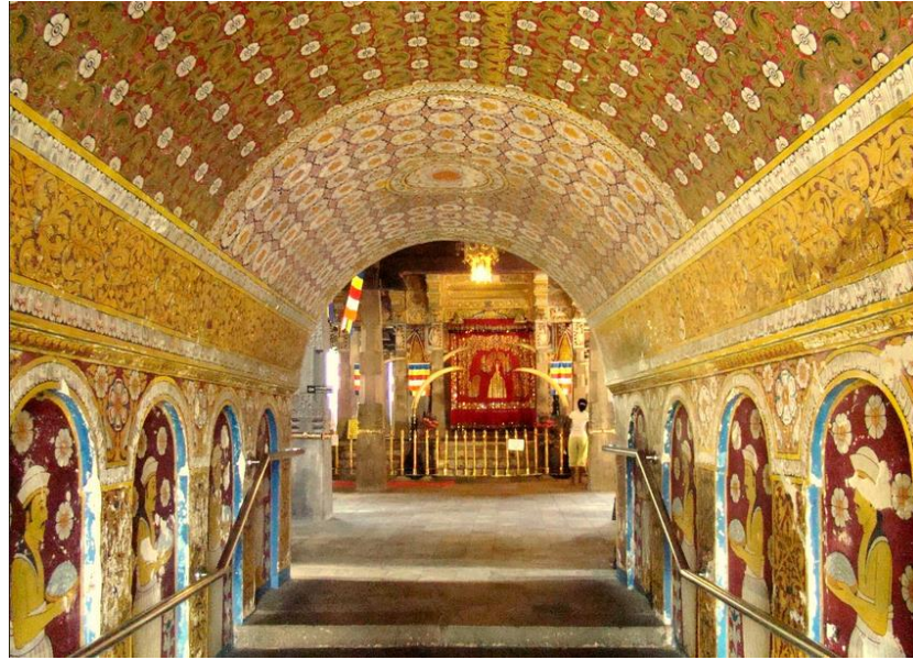
Figure 2.4: Barrel vault in Dalada Maligawa, Kandy.
