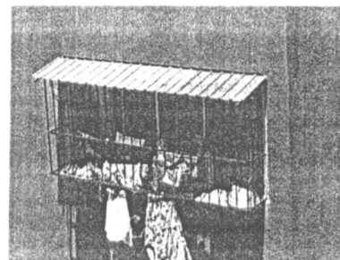
Fig 3.46: Projected store room at rear balcony
