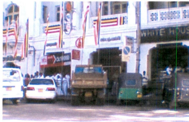
Fig 82 : Active building front of Kodituwakku Building; Dalada Veediya
