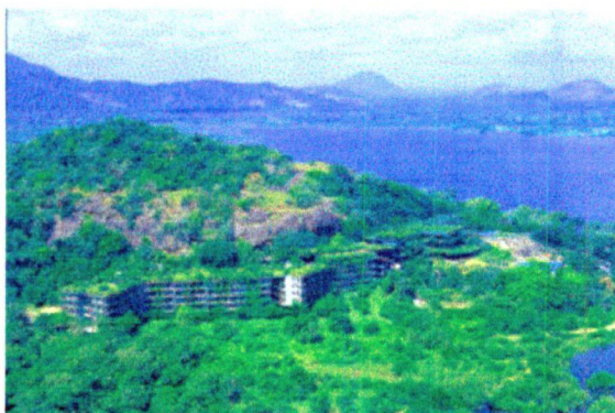
Plate. (61) Composition of the building form with the whole context The resultant form as a whole well balanced with the context, as a horizontal strip which running around as a continuing band.
