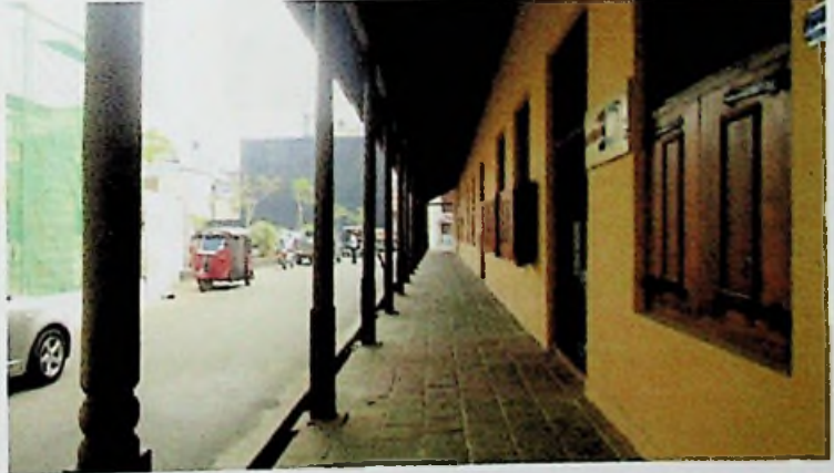
The entrance varendah facing the hospital street
