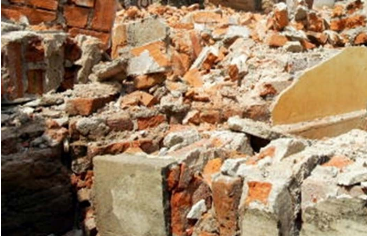
Figure A15.3: Brick Debris
