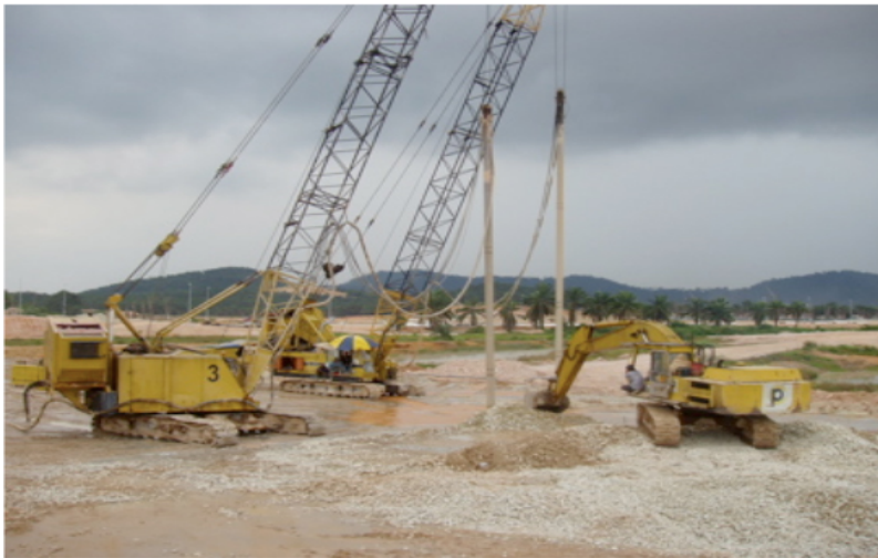
Figure 1.1: Aggregates Usage in Stone Columns in Road Construction ( www.waikogroup.com )
