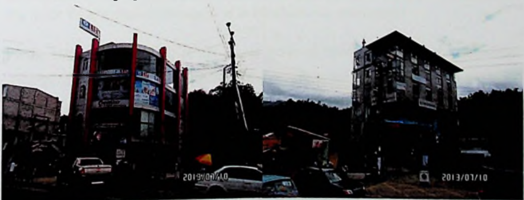
Fig 4.19: Utility lines creating disturbances
