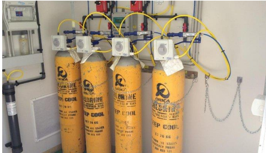
Figure 4.8: Conventional gas chlorination arrangement
