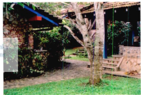
The residential zone. The making of a place that suits the childhood- a manifestation of the correct combination of color, texture and so forth. Fig:51
