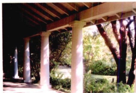
The more will be the openings the lesser will be the presence of a defining plane. Fig:31
