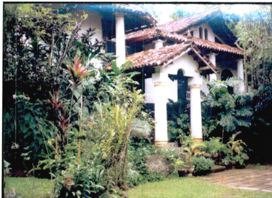
Figure 57: Front view of the house
