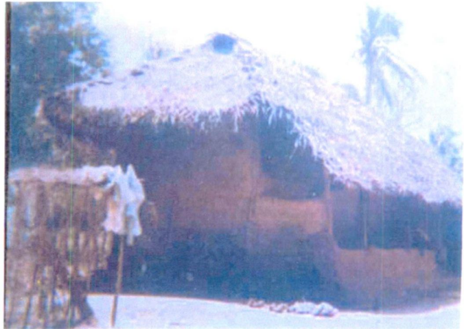
Figure 23 : Protection from sun & rain with large overhanging roof
