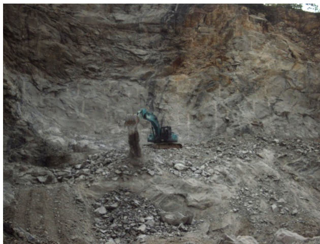
Figure 2.10: Mucking Using an Excavator
