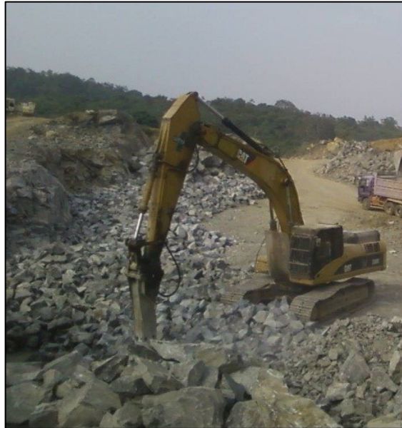
Figure 2.11: Rock Breaking
