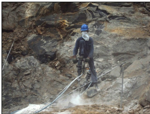
Figure 2.6 Left: Manual Drilling Using Pneumatic Hand Drill Machine Right: Mechanized Drilling Using Track Drill Machine
