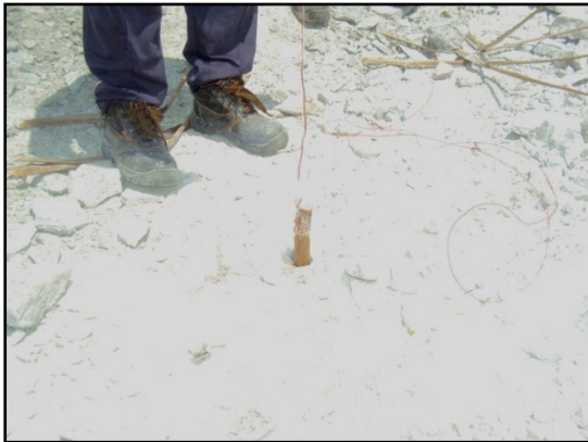
Figure 2.8 Left: Charging of Dynamite with ED (Primer)
