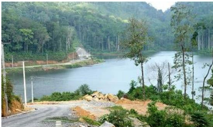
Figure 1.10 - Regulation Pond of the Kukule Ganga Hydro Power Plant
