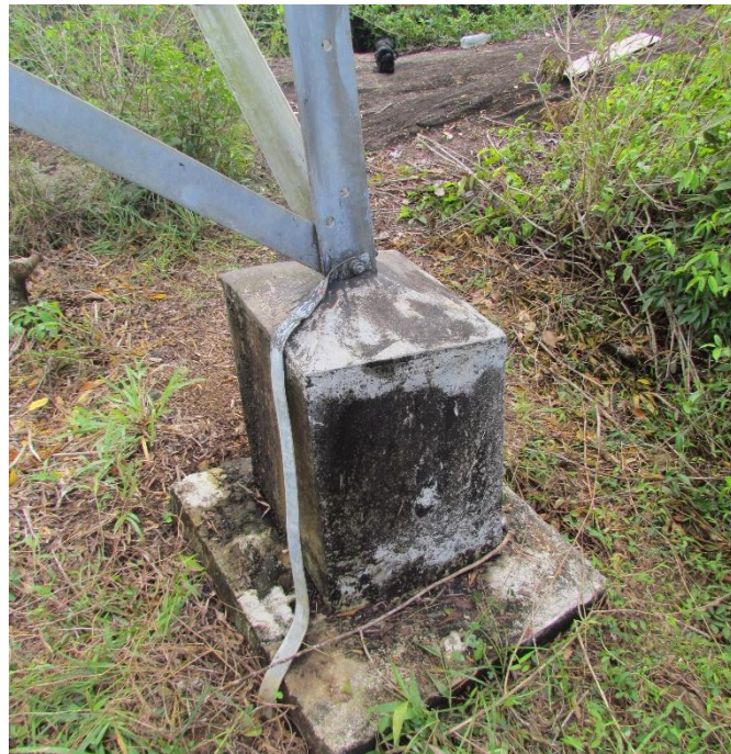
Figure 1.13 - Tower footing condition of the Tower-09
