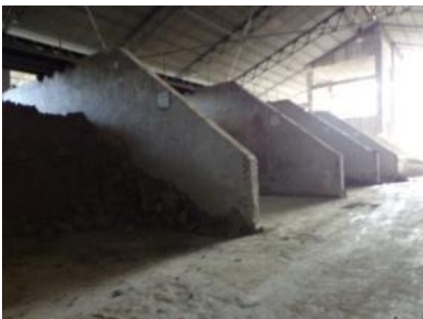
Figure 2.11: Raw material storage
