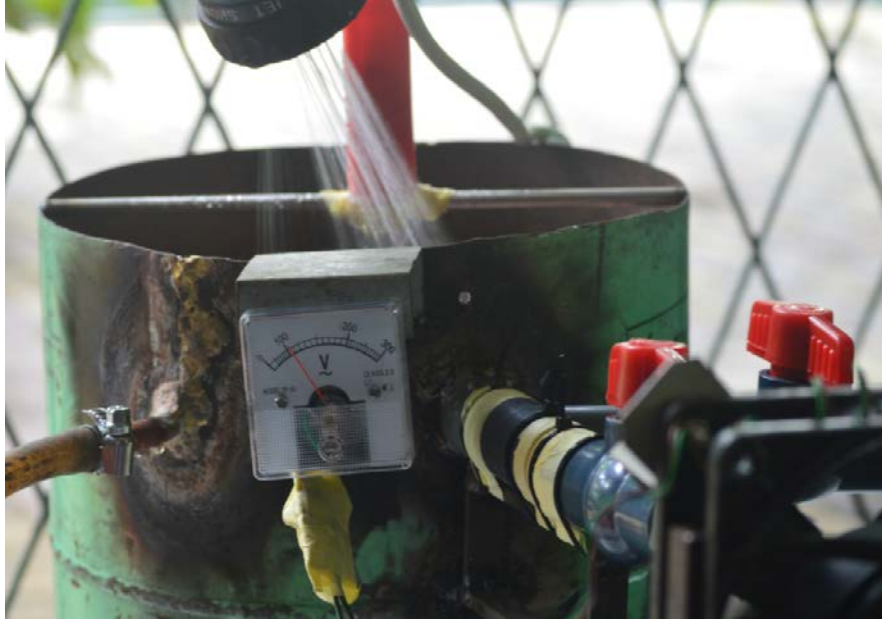
Fig 4.17 Water filling to heat exchanger
