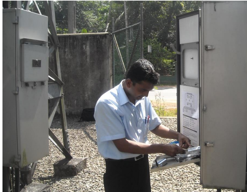
Figure 5.5: Installation of GPRS Modem
