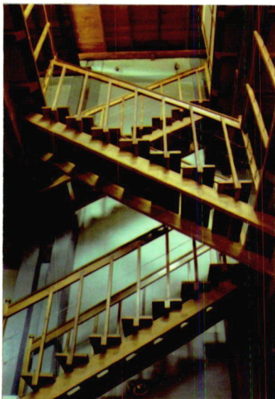
Plate-100-Stair way, Timber House
