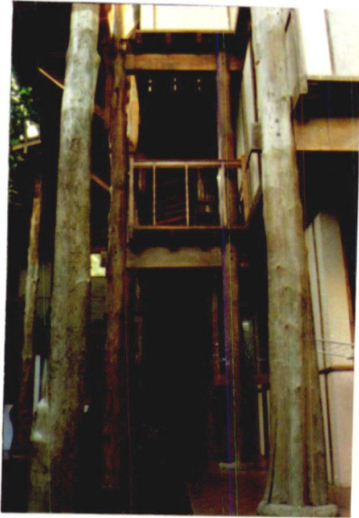
Plate-108-Columns, Timber House
