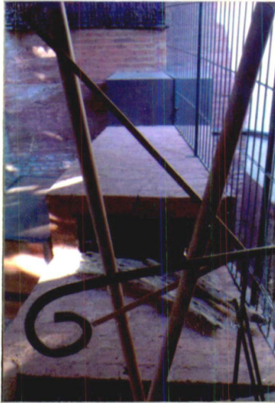
Plate-82-Detail, Steel House
