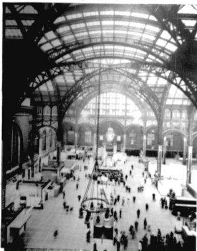
Plate 29- Pennsylvania Station, New York. USA
