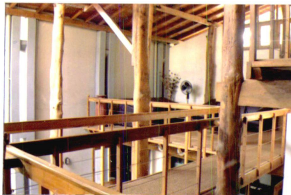
Plate-104-Living, Timber House
