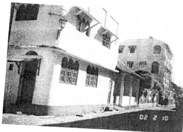
Fig: 4.35 – some of the buildings in Church Street
