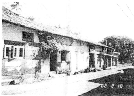
Fig: 4.30 –New buildings in Galle fort
