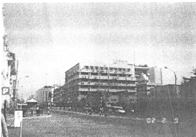
Fig: 4.10 - Eastern side of the York street
