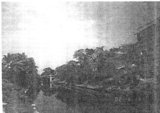
Fig - 29 Galle road bridge - Wallawatte canal
