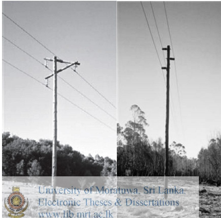
Figure 4.3 Traditional design (L) and new design(R) of pole top assemblies
