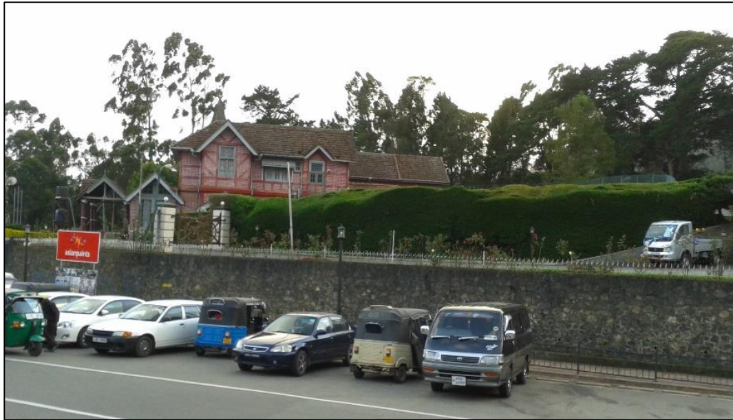
Figure 1.1: RRM Retaining Wall in front of Nuwara Eliya Post Office
