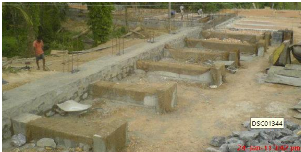
Figure 2.3 : Construction of Tie back arrangement at the site
