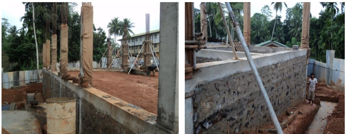
Figure 2.4 : Wall Foundations at the Rear Side of the Class Room block
