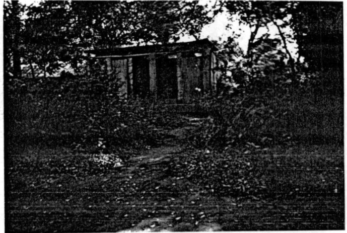
Fig. 52 Common sanitary facilities by local government, Mahakvekada, Kabithigollewa.
