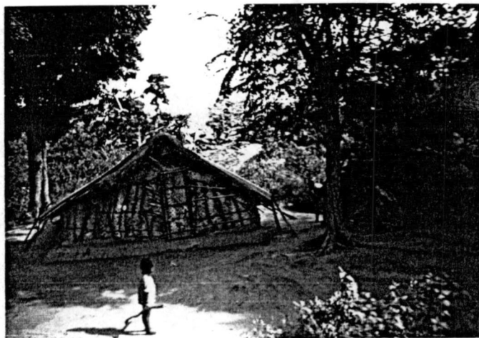
Fig. 45 Temporary hut out of coconut palm leaved panels. Resettled village, Morawewa.
