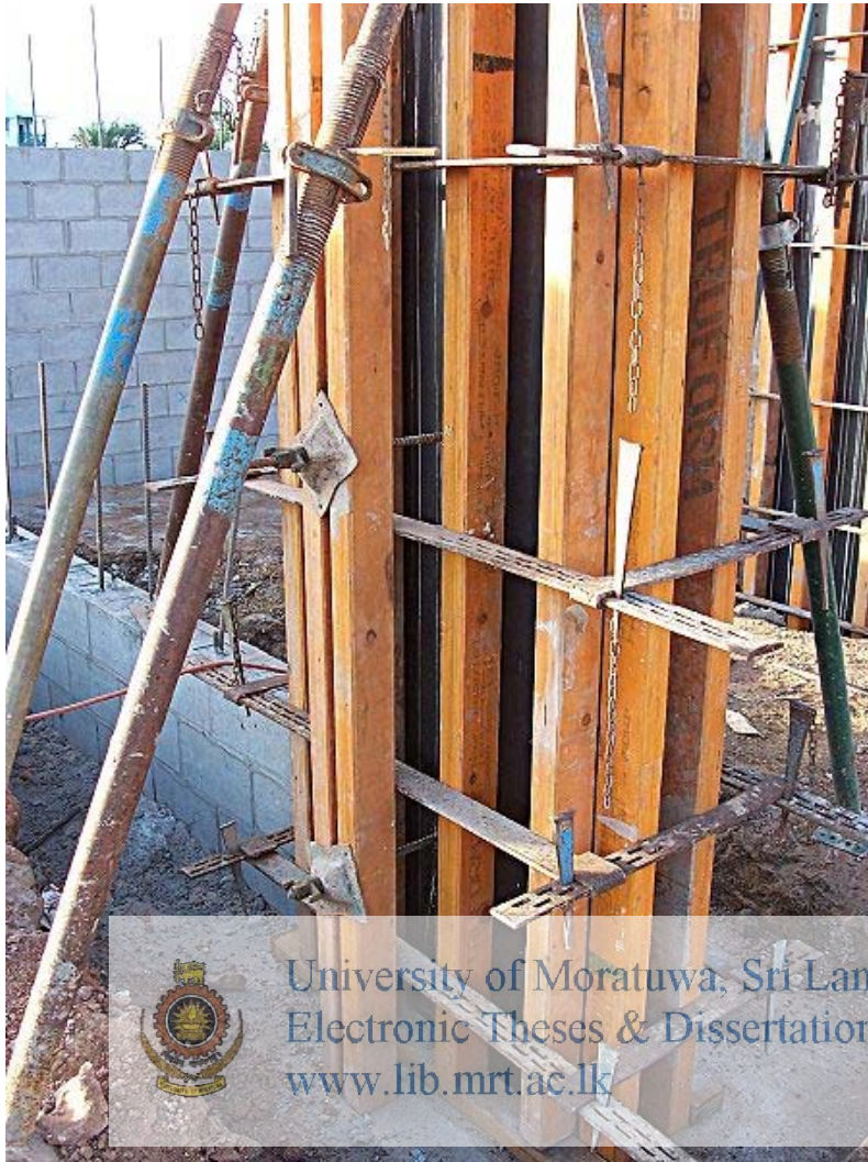
Figure 05: Modern conventional formwork for a concrete column
