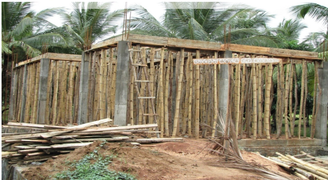
Figure 02: Conventional type formwork
