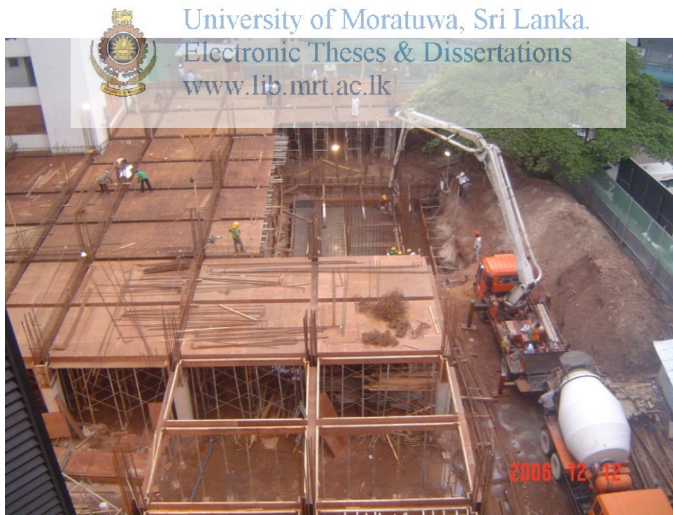
Figure 07: Modern conventional formwork for a slab
