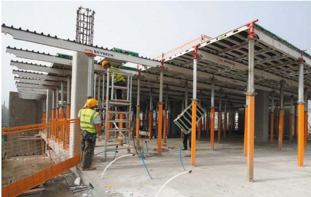
Figure 12: Typical system formwork
