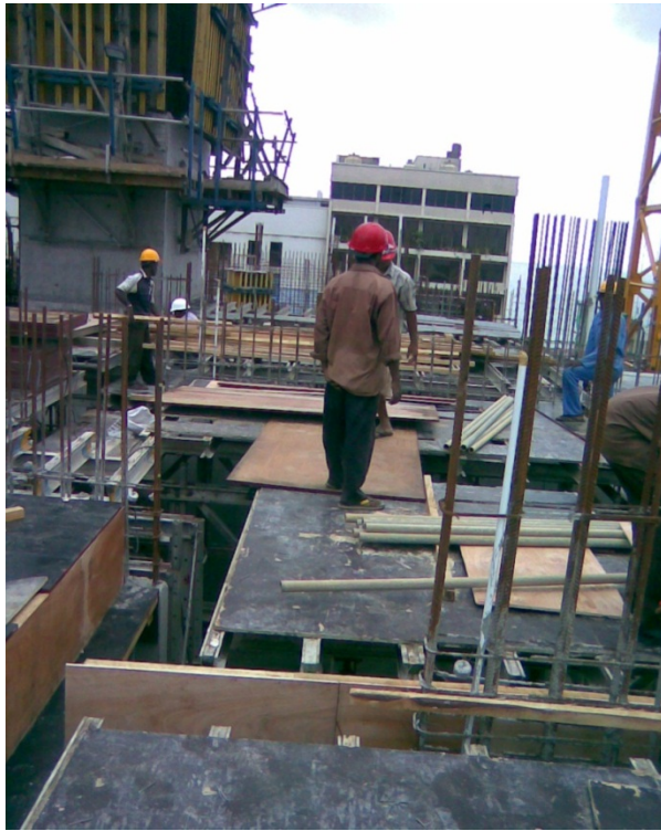
Figure 08: Modern conventional formwork
