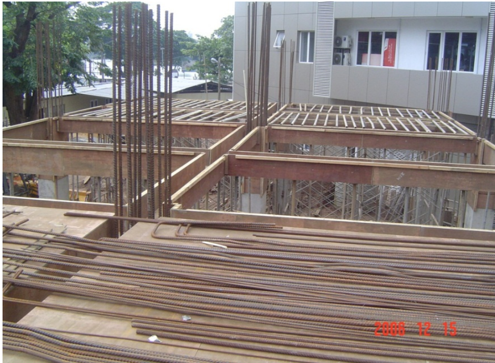
Figure 06: Modern conventional formwork for slabs and beams
