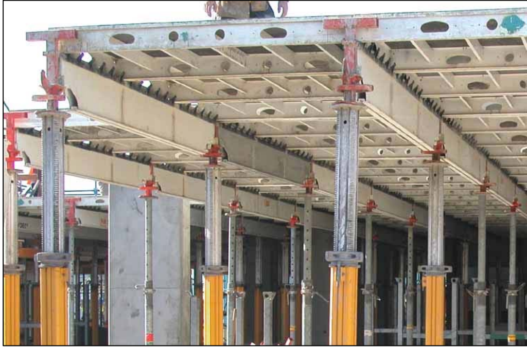
Figure 14: System formwork
