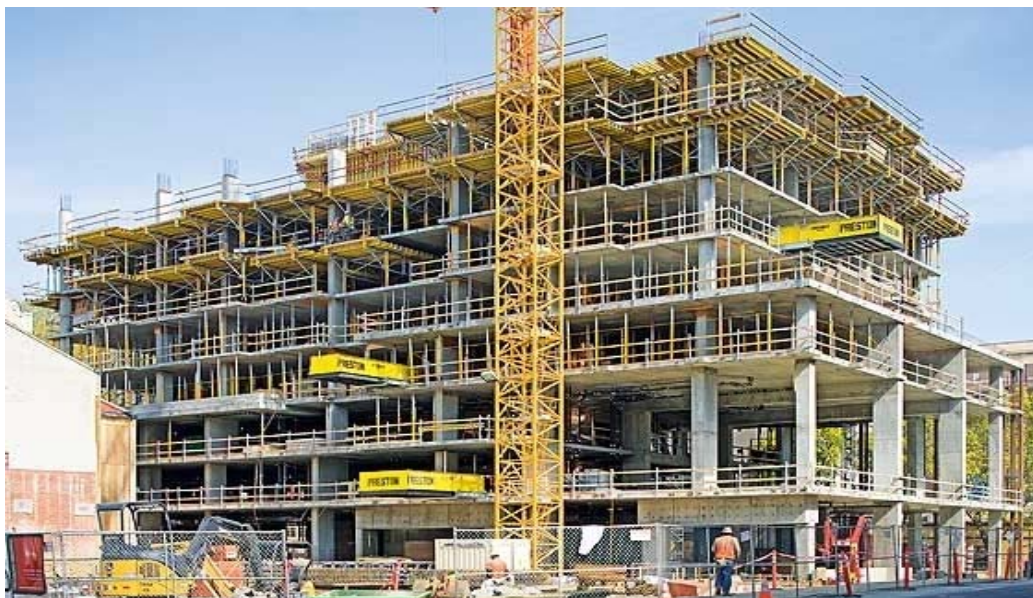
Figure 11: Semi-system formwork
