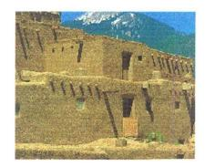
Figure 5 – Small openings located in solid walls reduce the heat penetration into the buildings
