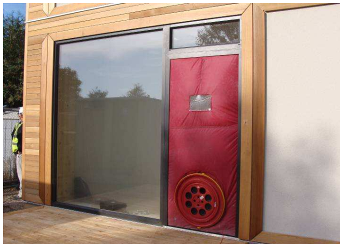
Figure 3: Blower-door fitted to the BaleHaus
