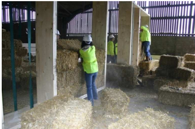
Figure 2: ModCell panel construction in a Flying Factory
