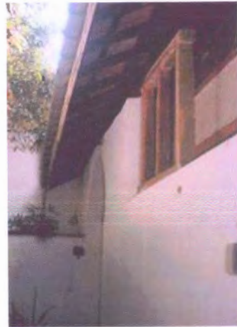
Fig51: Reuse window frame as a structural support
