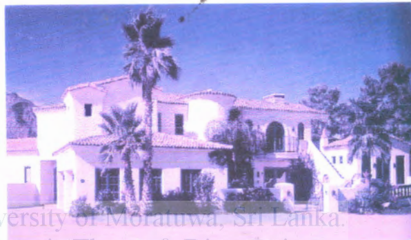
Fig06: the visitor center made out from recycled Styrofoam and concrete Source: Good house book
