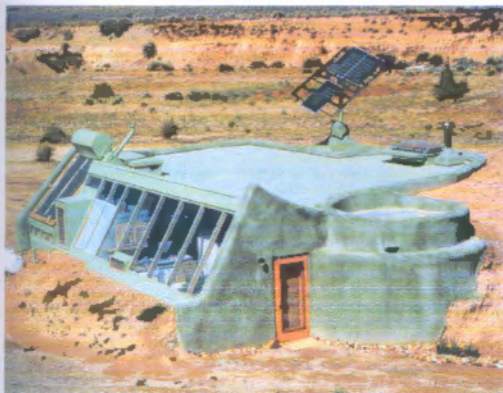
Fig 01: Earthship: the buildings' exterior walls are made mostly of used tires stacked and tamped full of dirt.
