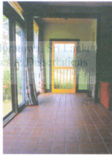
Fig:21 In winter on a sunny day the deep red tiles are bathed in sun and collect heat, preventing overheating during the day and slowly radiating heat into the room after sunset.
