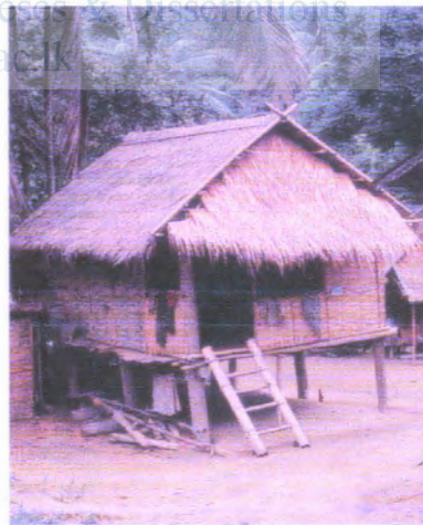
Fig12Grass house: large overhangs for the shade, permeable walls and free ventilation beneath the floor all the contribution to keeping this building cool in hot season.
