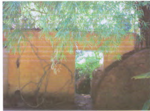
Figure 48: The entrance door The entrance arch made out from mud and bamboo strips
