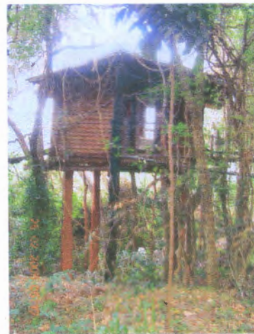
Fig 35: traditional 'pala' retain on the timber pillars
