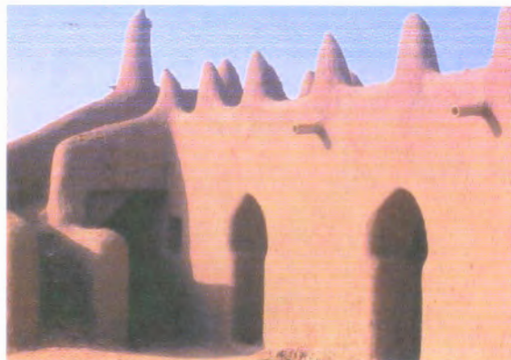
Fig18 Traditional adobe; thick thermal mass walls absorb solar heat, slowing its movement toward the interior. This building is in sanosa, Mali Source : www.kleiwerts.com
