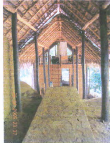
Fig:39 high pitch roof retain on the reused light post columns. Wide corridor focus on to viewing decks.
