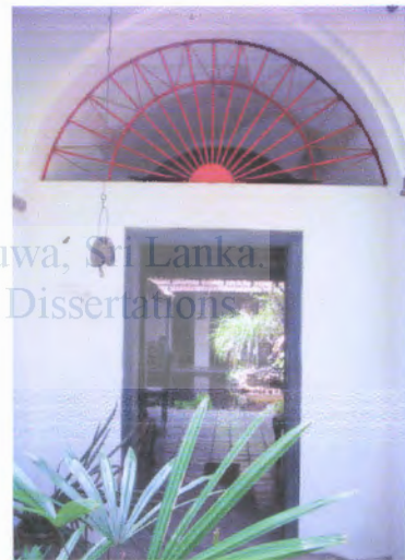
Figure49: the entrance door steel grill work prepared by reuse steel
