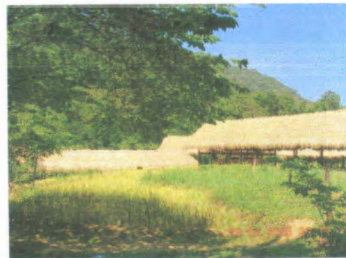
Fig40: 'illuck' thatch roof is the dominant feature of the Ella Adventure park
