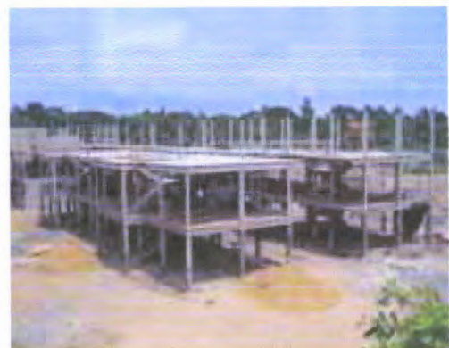
Fig59. construction of Don Bosco apartments Nigambo
